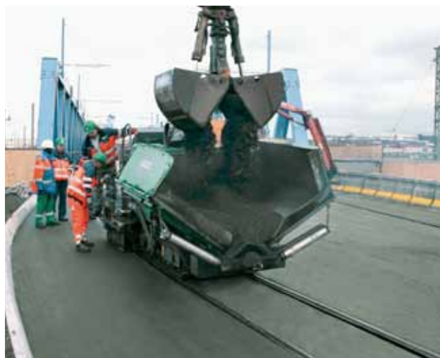
Paving asphalt between tramway tracks
