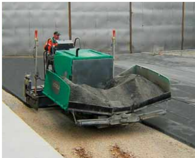
Surfacing large areas
